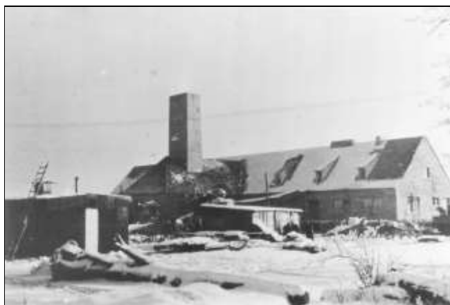
The almost finished Crematorium II.
